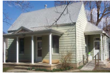
The Hannah Haines Brown Whiting and Horace B. Perry Home 727 South Main Street Mapleton, Utah
